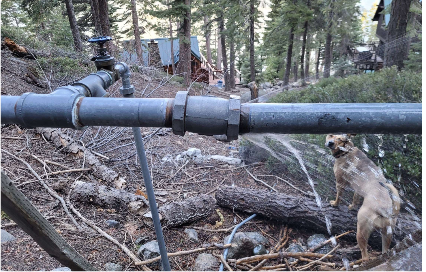
Not much of an offset in the pipe, but just look at the spray.
